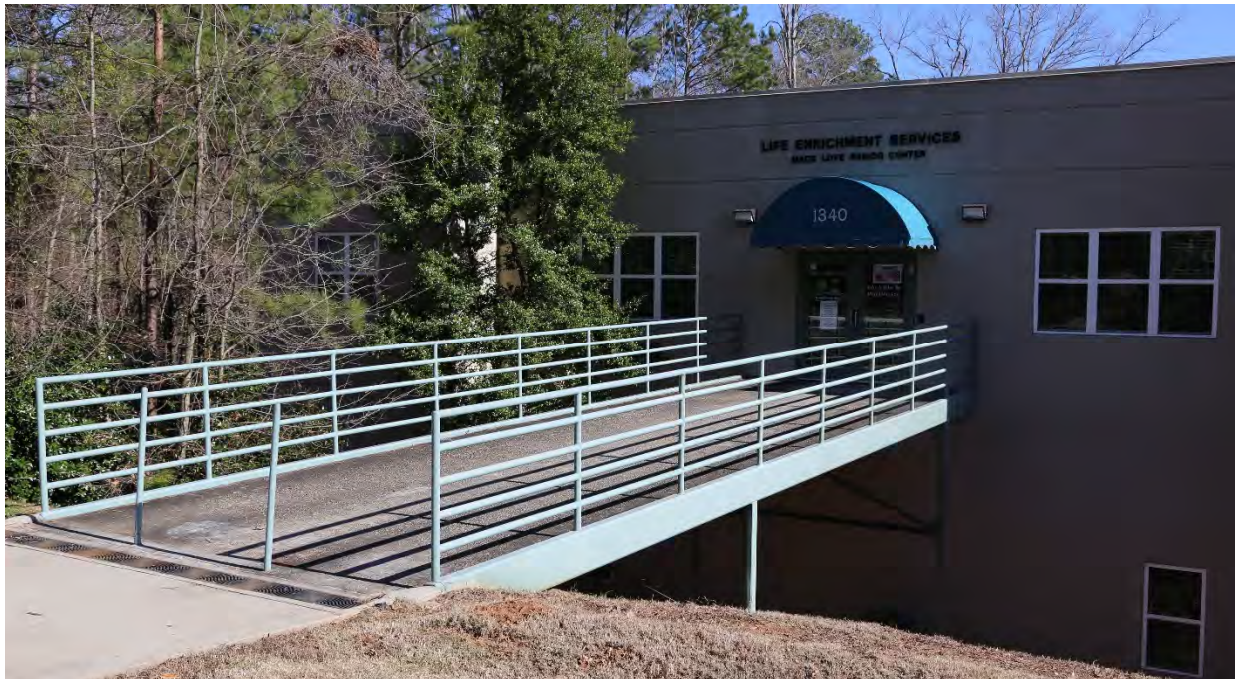
The second floor of the building serves as the Mack Love Senior Center (Life Enrichment Services) and is accessed from the south elevation on McConnell Drive.
