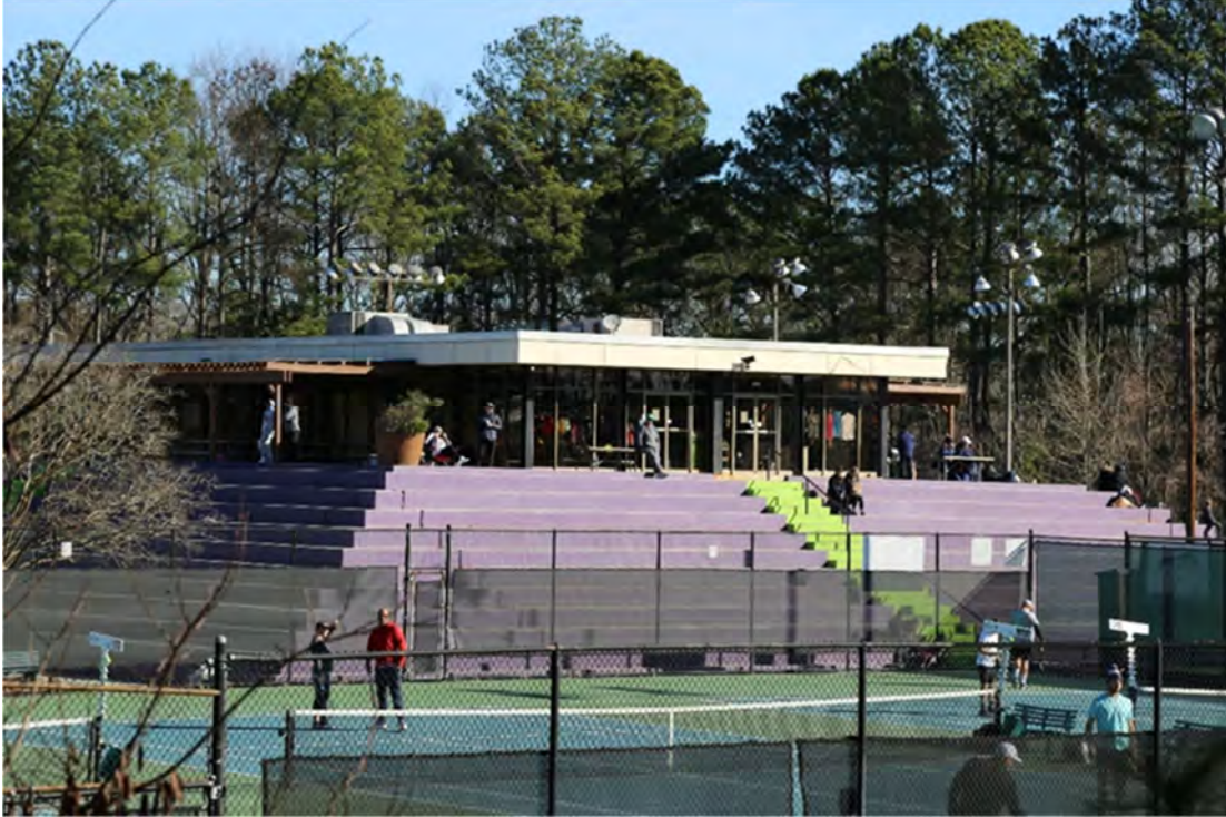
View of the existing tennis pro shop atop tiered concrete ziggurat
