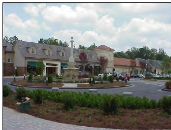
Example of commercial development, The Forum in Norcross, GA
